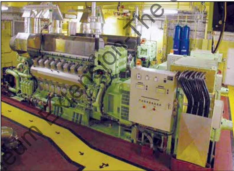
Figure 1. Large internal combustion engines power drilling rigs.
