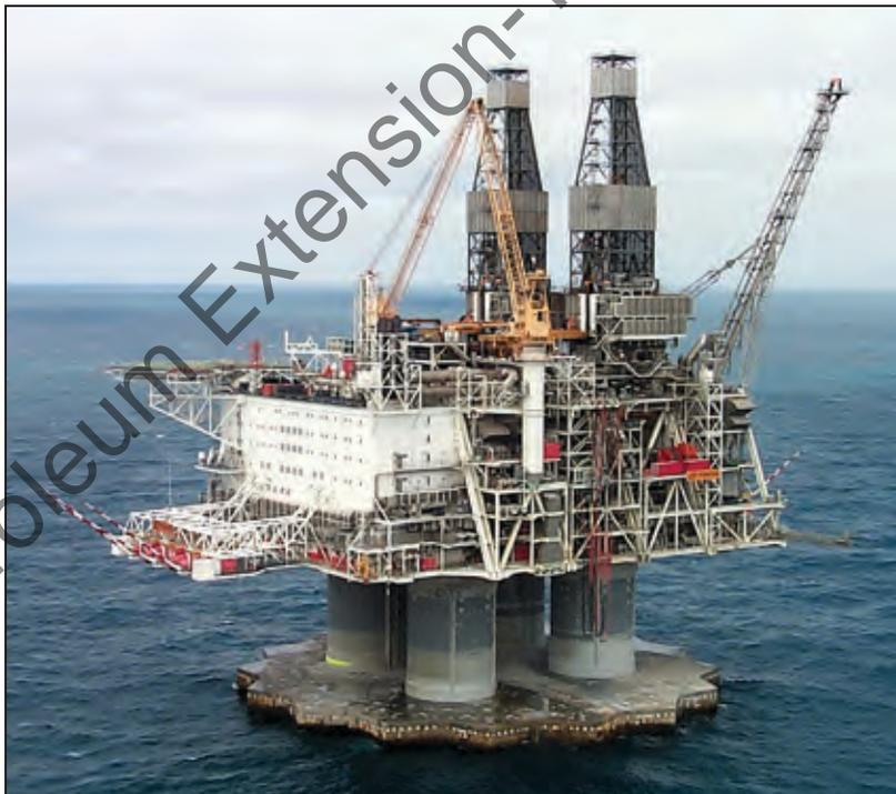
*Figure 3-2.1. This self-contained platform, the Hibernia, houses all the drilling and production equipment and facilities for the crew. The Hibernia is located off the coast of Newfoundland and is the world's largest oil platform in terms of weight.*
