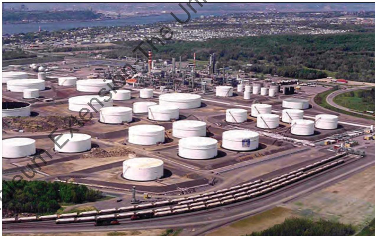
*Figure 4-2.1. A refinery is an organized and coordinated arrangement of processes (called units) linked together with miles of pipe carrying crude oil in and products out. Pictured: Valero Corporation's Jean Gaulin Refinery in Quebec, Canada, has a capacity of 215,000 barrels per day.*
