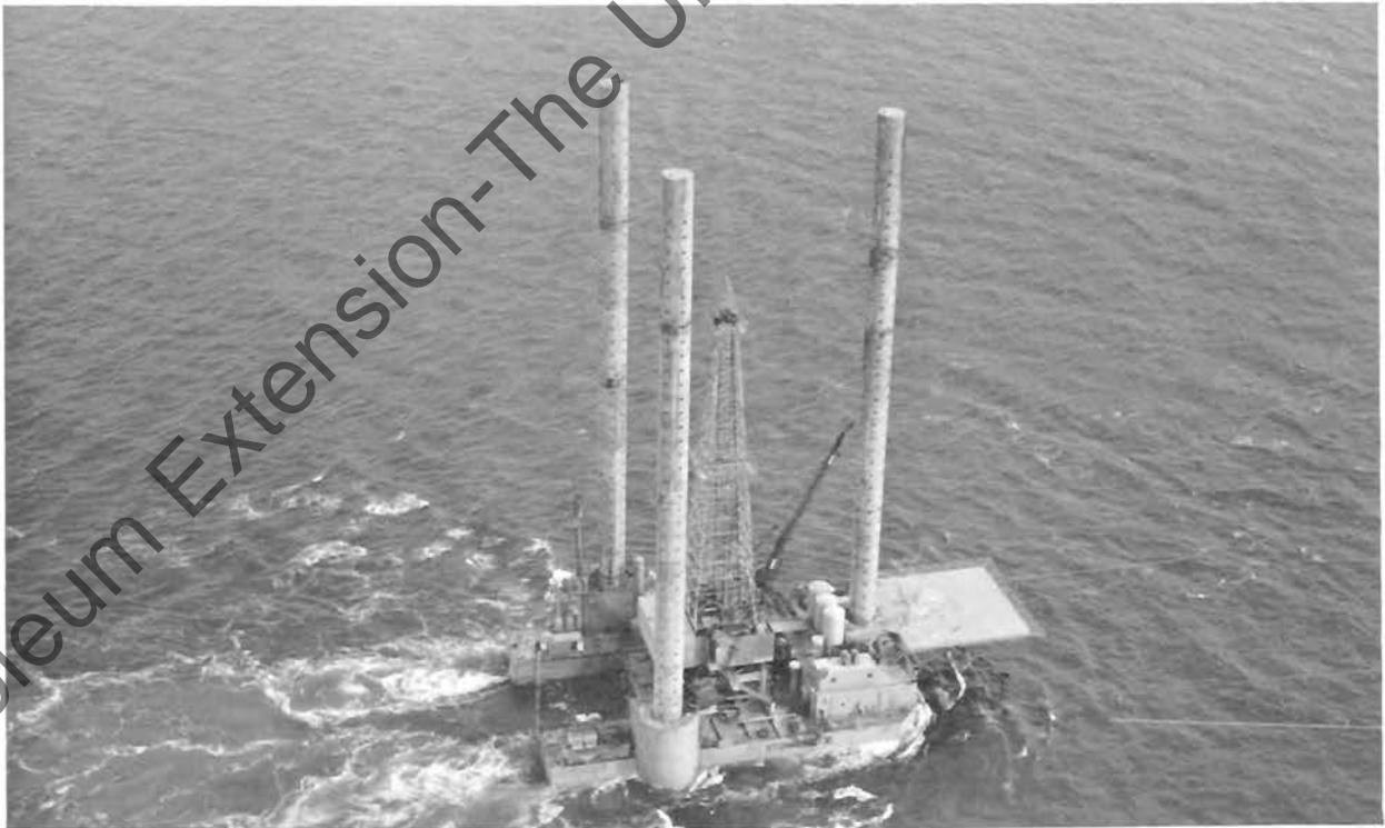
Figure 19. Mat-type drilling unit under tow
