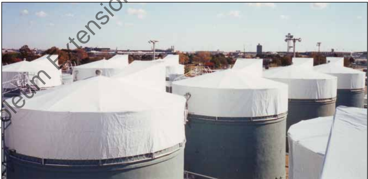
Figure 12.1 A top view of a tank battery
